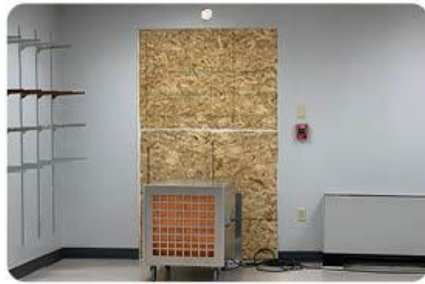
Figure 3, Med/Surg Soft Wall and Negative Air System.
